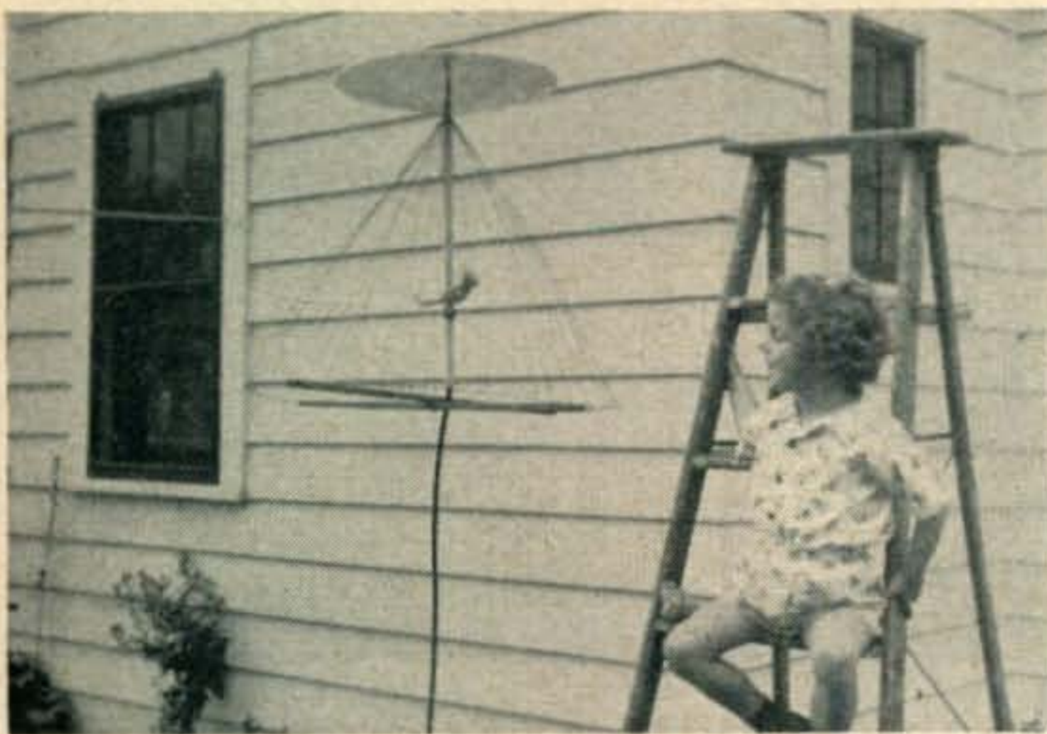
Fig. 3. The 100-mc discone, as arranged for photographing by the jr. op, Susie. The aluminum disc is 20" in diameter, and the 60° cone is formed of 48 wires, each 37" long. This bird cage is permanently installed in the attic and is used mainly for 2-meter work.
